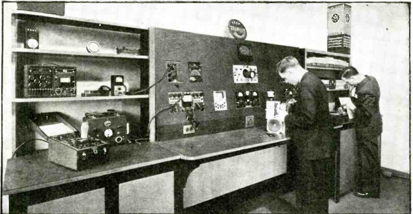
Fig. B. Interior view of the Model Service Shop of the Radio College of Canada, showing highly efficient arrangement of test bench and equipment.
